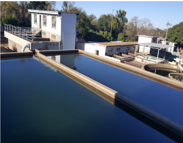
Bela- Bela Water Works
